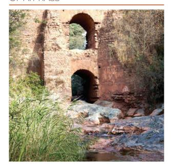
Traditional historic bridge, located between the 2 banks of Oued Mhasseur, integrating in its structure arches for the passage of floods. Location: right next to the Imin'lfri site.
